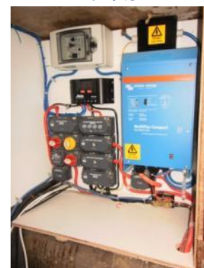
Complete new shore power system fitted.
