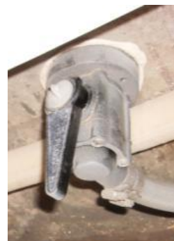
New fitted Marelon valves.
